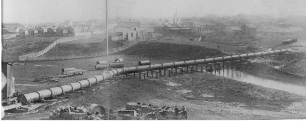
A water line extension built in the late 1800's – photo courtesy of Louisville Water Company
