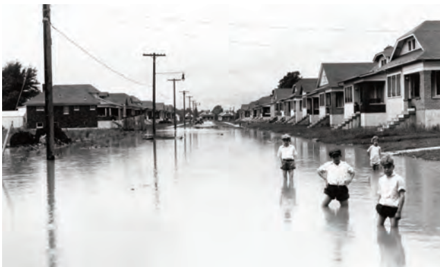
A branch of Mill Creek flooded Manituva Avenue, newly constructed without drainage infrastructure, in 1929.
