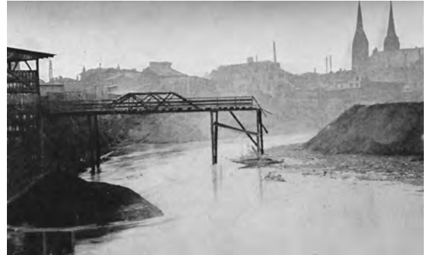
Packing houses routinely dumped offal into Beargrass Creek where it ran through Butchertown. High water after a snow melt partially collapsed a bridge constructed to allow dumping on both sides of the stream."
