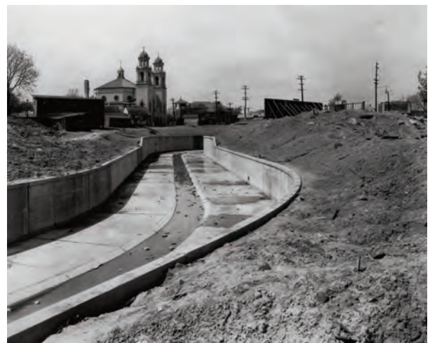
Trying to control flooding, the South Fork of Beargrass Creek was converted into an engineered channel, with a dry-weather channel running down its center.
